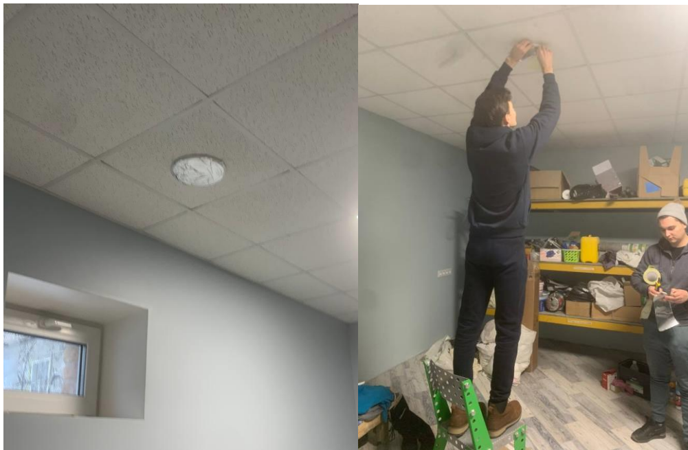
Fig.6.7 Ventilation sealing
