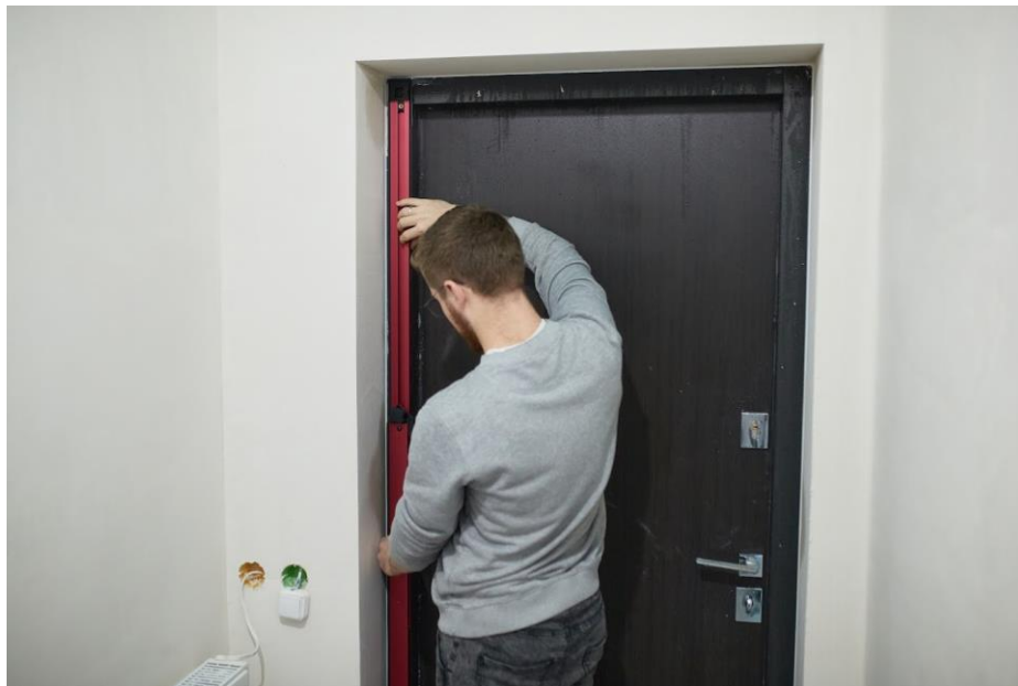
Fig. 6.9 Adjusting the height of the door frame
