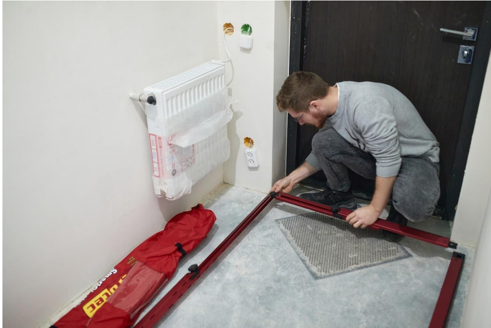
Fig.6.10 Assembling the air door
